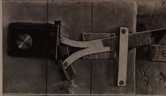
Sliding Doors Fitted with This Spring-Type Lock Provide Additional Security to Either Garage or Barn
